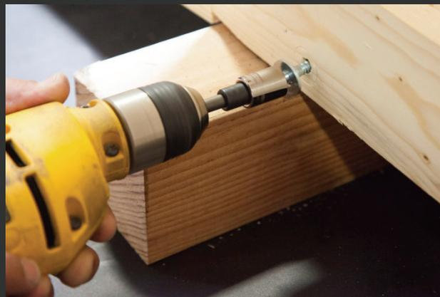
Using a  $\frac{1}{2}$ " socket bit with either a wrench or power drill, remove 3 bolts from the bottom of each of the three remaining sides of the crate. (9 total)
